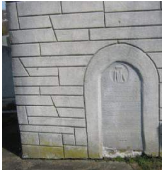
Outside back wall
